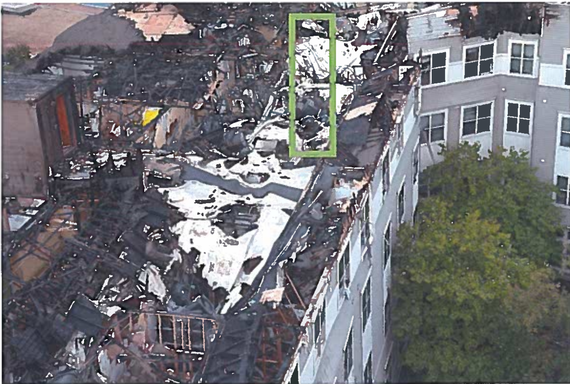
Garden Hose Pulled Towards Area of Origin
