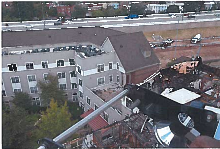
Undamaged Roof Section on “BC” Corner
