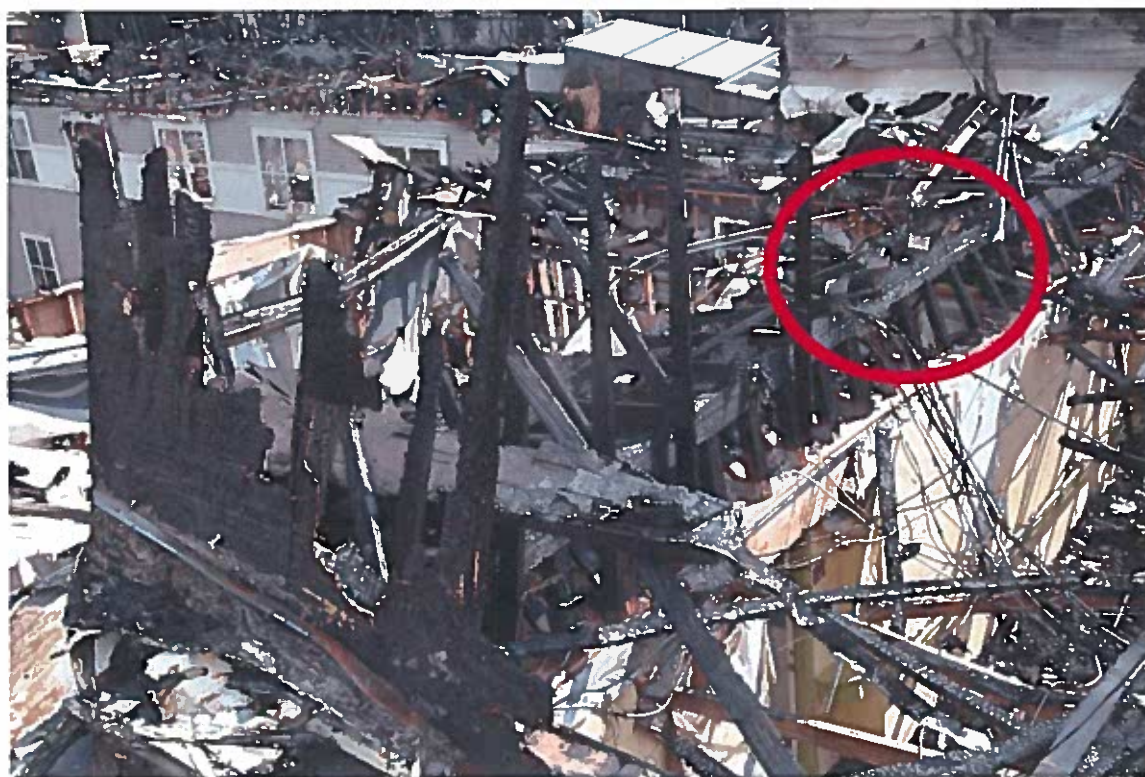
Area of Origin in the Cockloft above the Kitchen for Apartment 431
