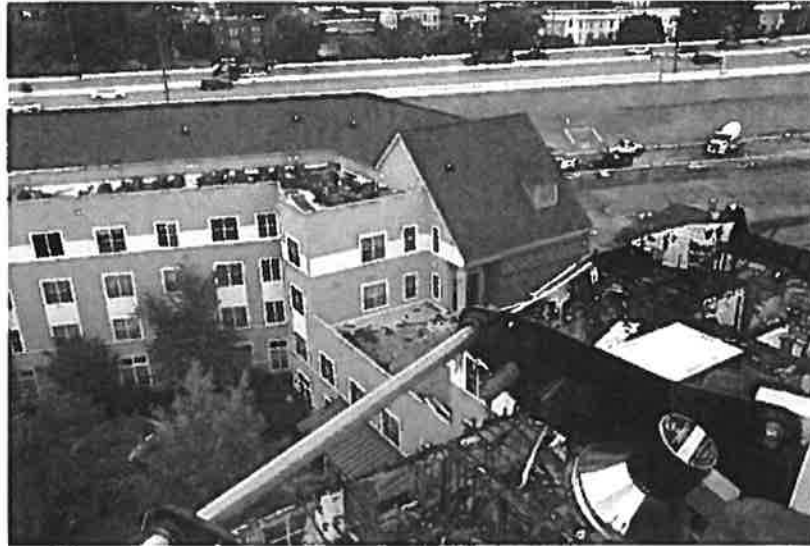
Undamaged Roof Section on "BC" Corner
